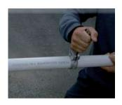
The PVC pipe cut should be completely straight to ensure that it fits perfectly inside the elbow. Avoid any unnecessary bends or deviations.
