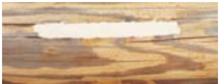
Cavity filled with E-Wood
